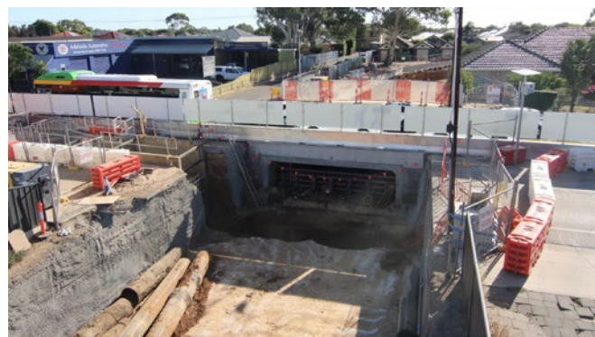
Marion Road Crossing Works
